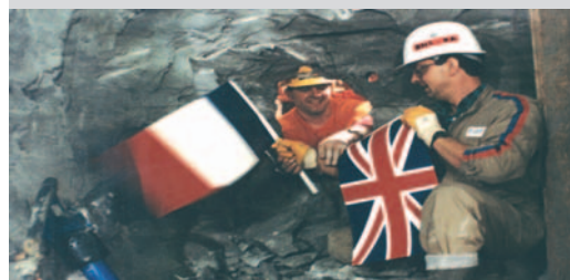
Break through – Eurotunnel
